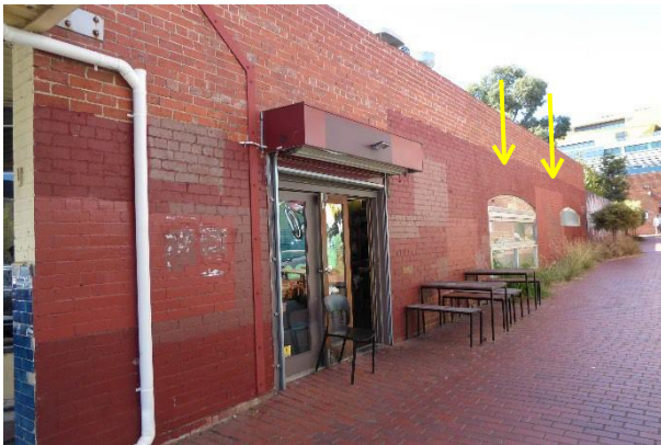
Alley – north side (18 Derby Road). Note original arched openings.
