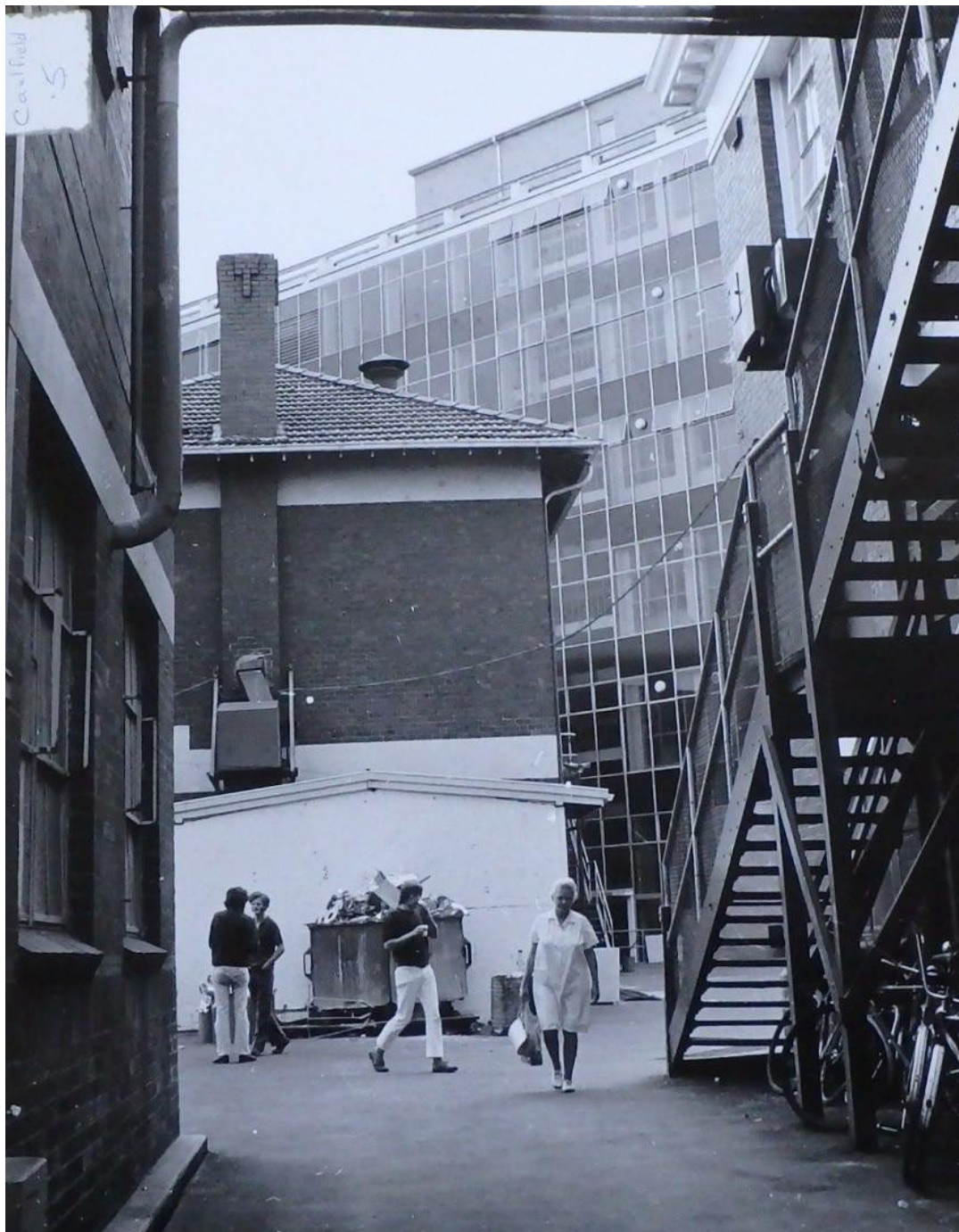
The southern elevation of the Diploma Wing, early 1970s – note the level of transparency to the curtain wall. (Source: PROV, VPRS2115, P0, Unit 6)
