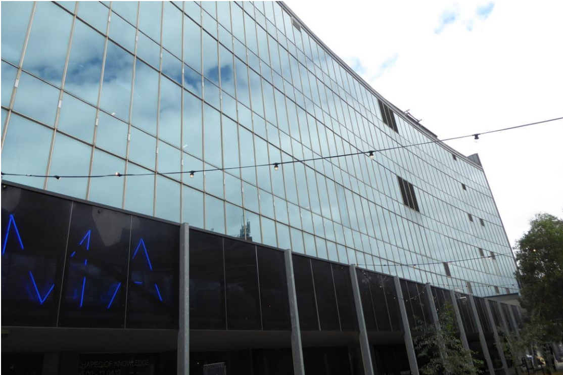
Southern elevation with canopy addition in the foreground.
