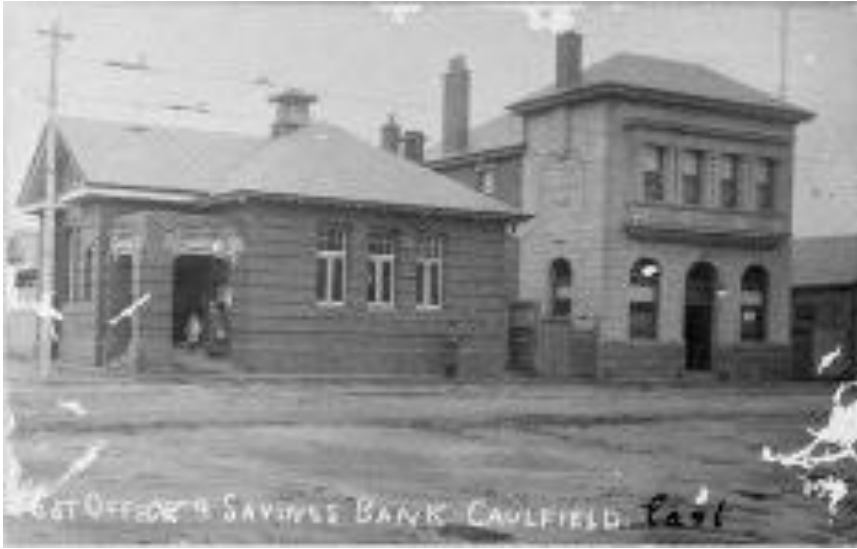
Photograph of Caulfield East Post Office (right) and State Savings Bank of Victoria (left), 1913-15. Note the introduction of the tram line to Derby Road. (Source: B5919, NLA)
