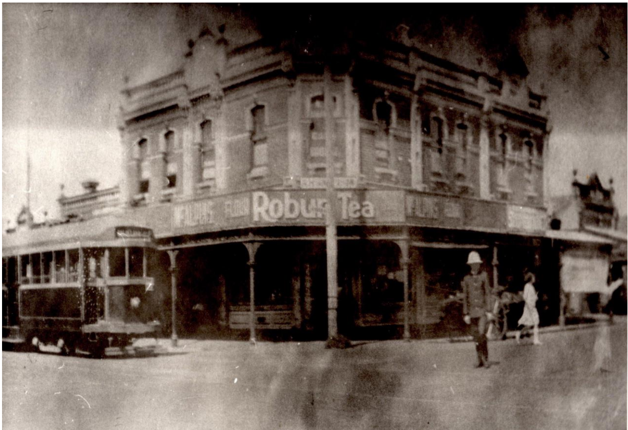
Early 20 th century photograph of Wybar's Building (HO91) at the south-east corner of Balaclava and Kambrook roads. The triangular pediment (and urns – since lost) and vernadach of Wybar's shop/residence at 26 Kambrook Road are visible right of frame. (Source: courtesy of Glen Eira Historical Society)
