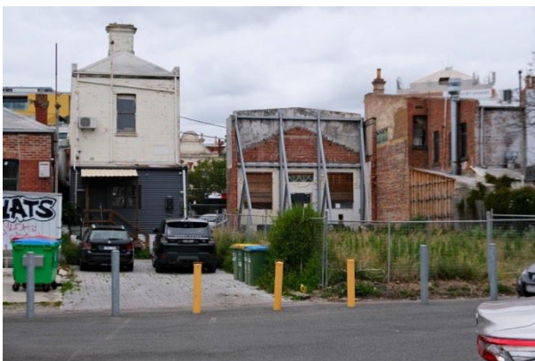
Rear of 7 to 15 Derby Road.
