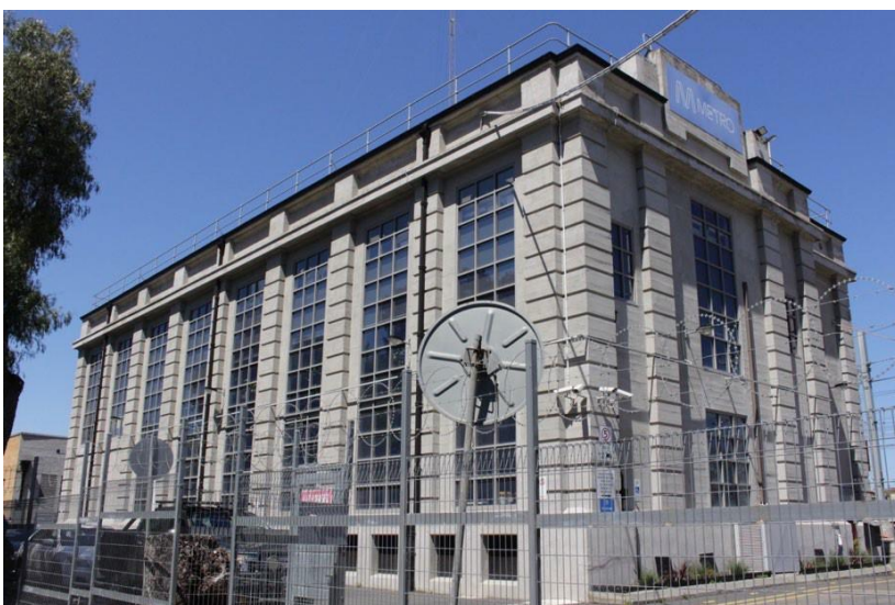
View to the northern (long) and eastern (short) elevations.
