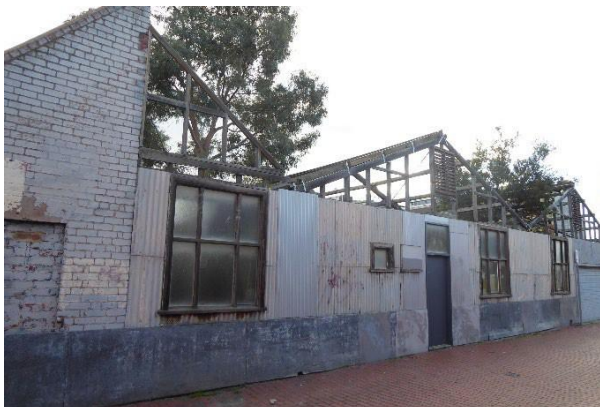
16-22 Derby Road. Likely original roof forms and window frames.
