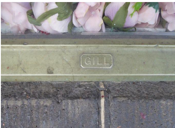
2 Derby Road – Gill shopfront band and basalt plinth.
