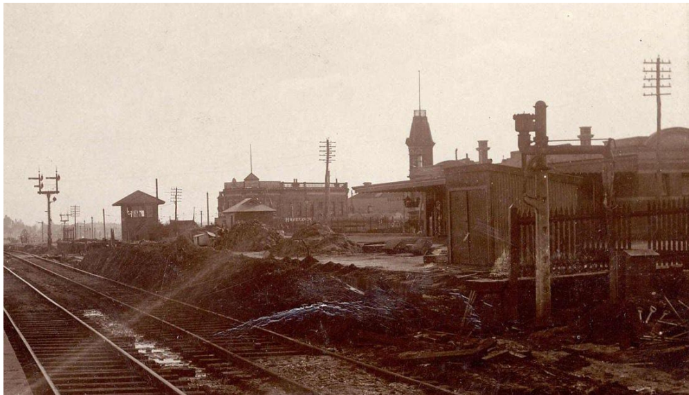
Photograph depicting rail work near the precinct, circa 1914 Note the original design and height of the tower at 2 Derby Road as well as the opposite parapet detailing at nos 1-7 (opposite) (Source: Caulfield Railway Station , SLV, H86.98/174)
