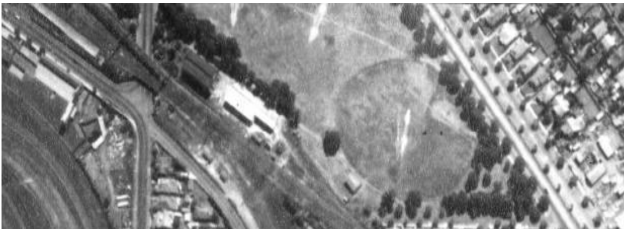
1956 aerial photograph of the Caulfield Railway Substation , identified by the red arrow, with construction depot/workshop present to the east. (Source: Melbourne Outer Suburbs Project , no. 250, Run 15, Frame 73, Landata)
