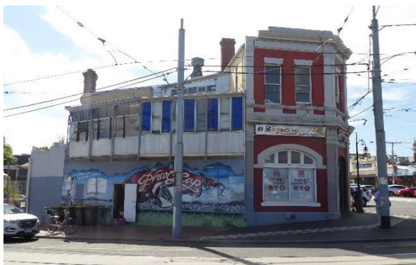
1 Derby Road in foreground, chimneys of nos 3-7 in background.
