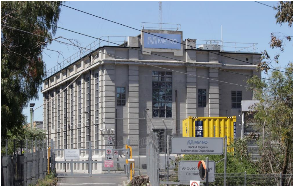
Queens Avenue frontage, showing the western elevation (short) and northern (long) face.
