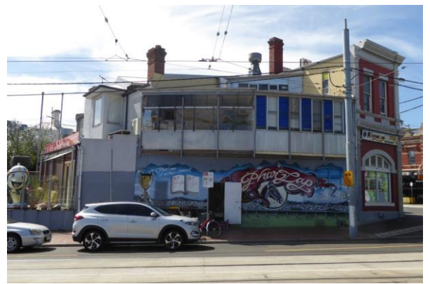
Side view of 1 Derby Road.
