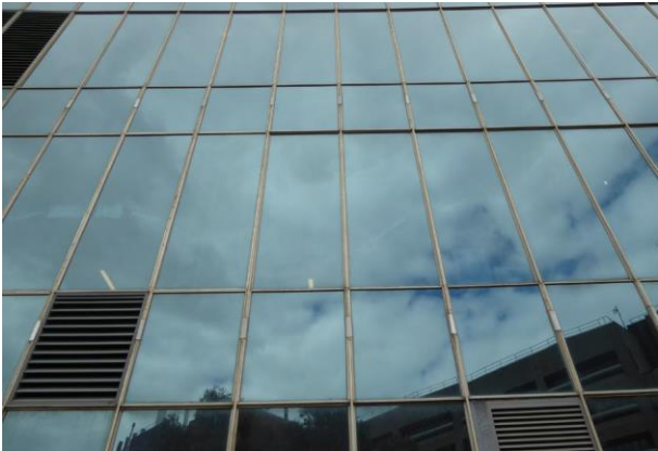
(Above) Detail of curtain wall, southern elevation.
