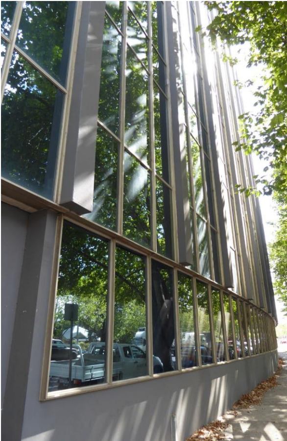
(Above) Detail of curtain wall, southern elevation.
