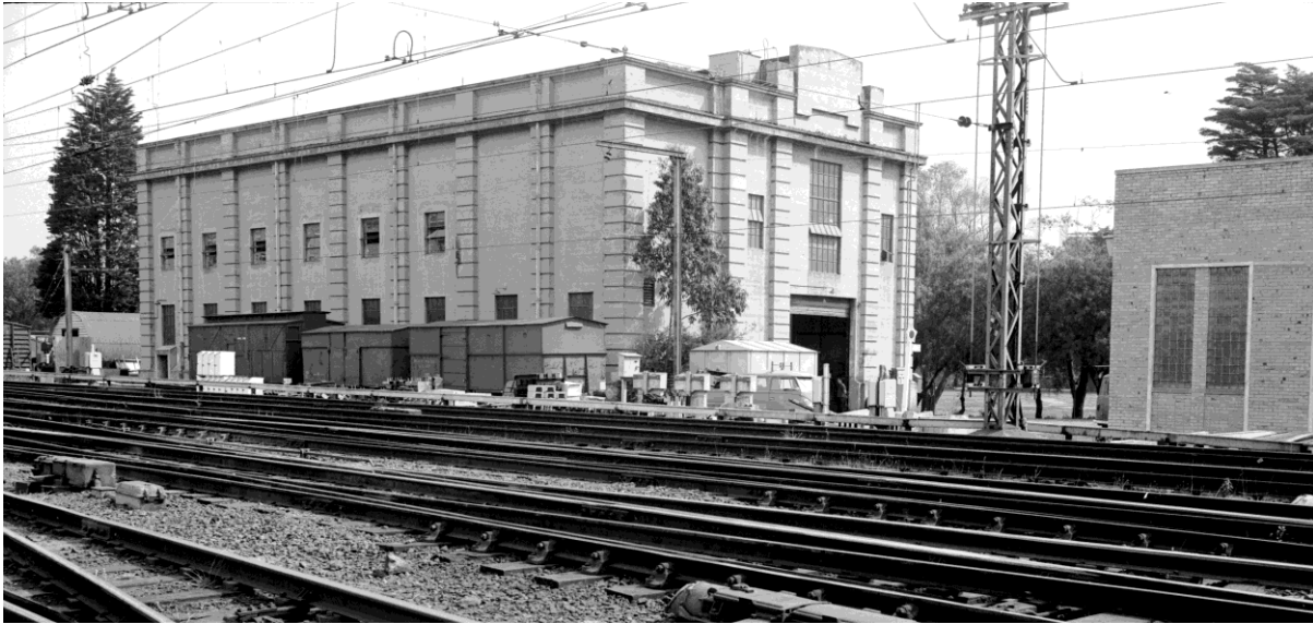
A mid-to-late 1950s photograph of Caulfield Railway Substation from the railway line and, to its right, the construction depot/workshop. (Source: Photographic Collection: Railway Negative: Alpha-numeric systems , VPRS 12800, S 1132, PROV)
