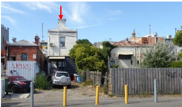
West side – rear of no. 17 (L), no. 15 (middle, highlighted), no 9 (R).
