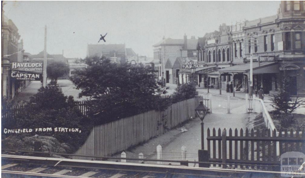
Photograph of Derby Road, facing north from the original subway, around 1913 Note the presence of since replaced timber buildings at nos 16-22 with gable ends (red arrow). (Source: Caulfield from the Station , Victorian Places website, John Young Collection)
