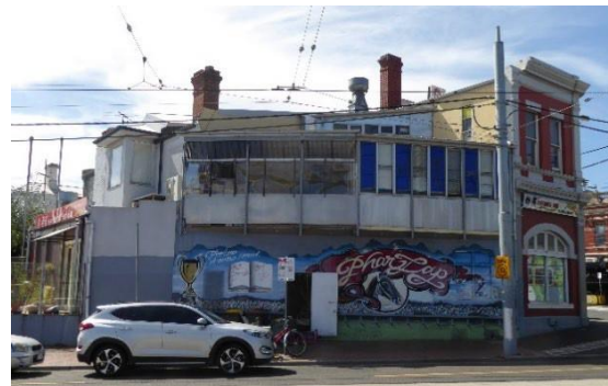
West side – rear of nos 1, 3-7.
