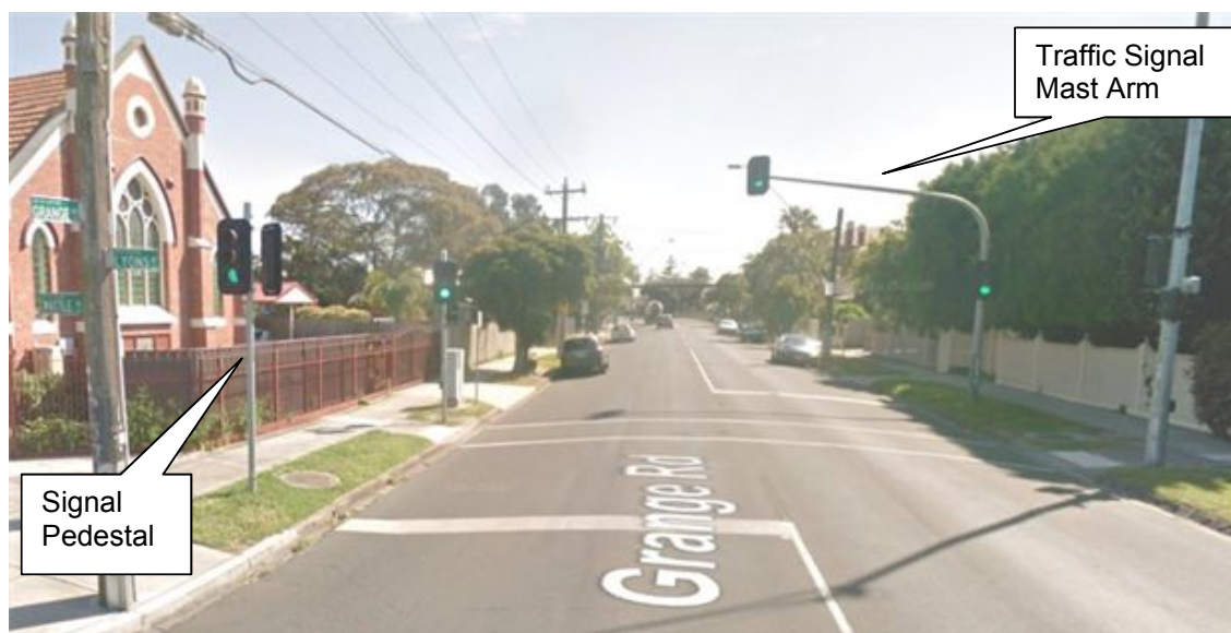
Grange Road Pedestrian Operated Signals (with mast arm)
