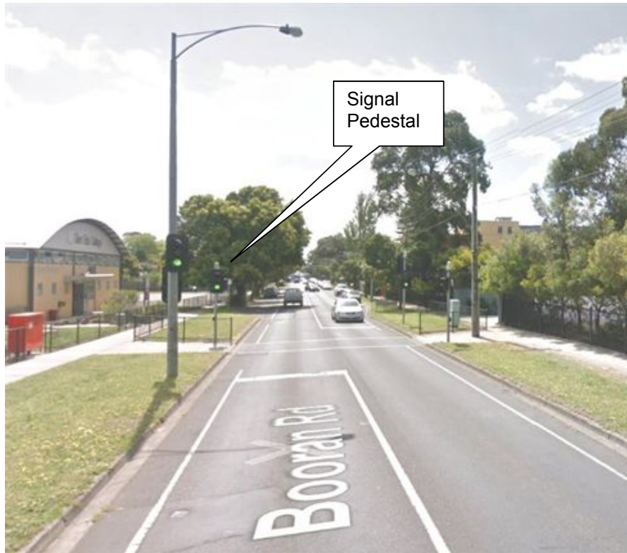
Booran Road Pedestrian Operated Signals (without mast arm)
