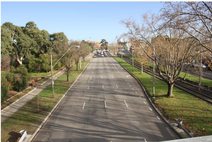
Existing road configuration in front of Alma Park.
