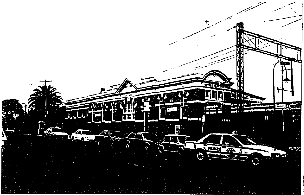
Platform 4 building: Railway Avenue
