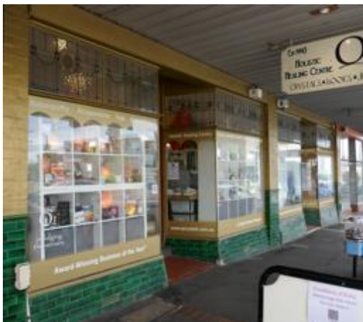
Figure 14. Early shopfronts including tiles, central in-go and stained glass highlights at 743-45 Glenbuntly Road. Source: Trethowan Architecture 2021.
