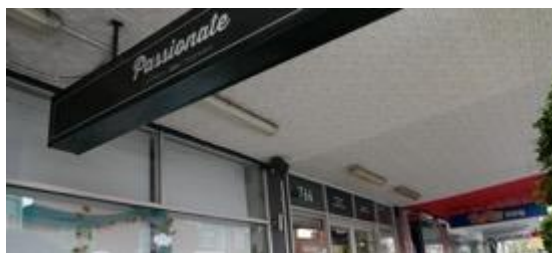
Figure 13. Detail of pressed metal soffit at 766 Glenbuntly Road. Source: Trethowan Architecture 2021.
